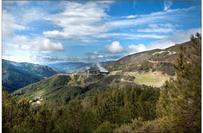
Calpine's Grant (Unit 20) at The Geysers. Photo by John Grice courtesy Calpine.
